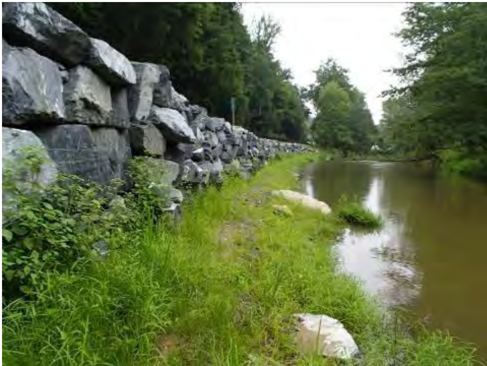
Removal site looking upstream along the left ascending bank at start of imbricated wall
